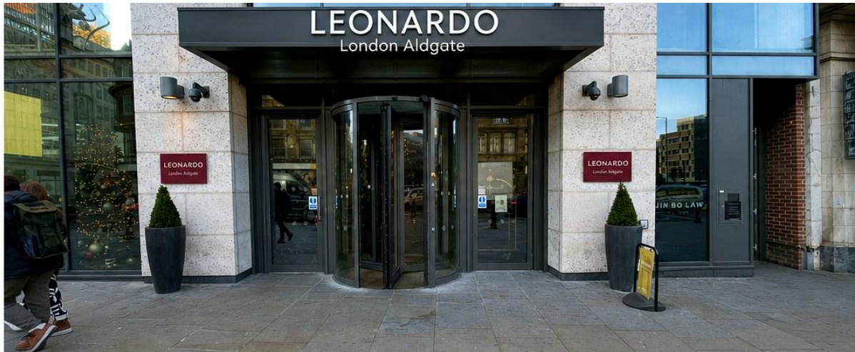
Accessible entrance doors located beside the revolving door, providing level access into the hotel.
