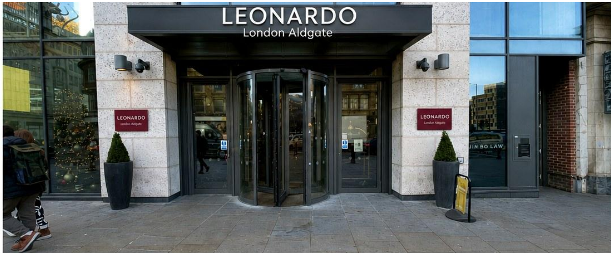
Main entrance showing the revolving door and accessible side doors with step-free access from the pavement.
